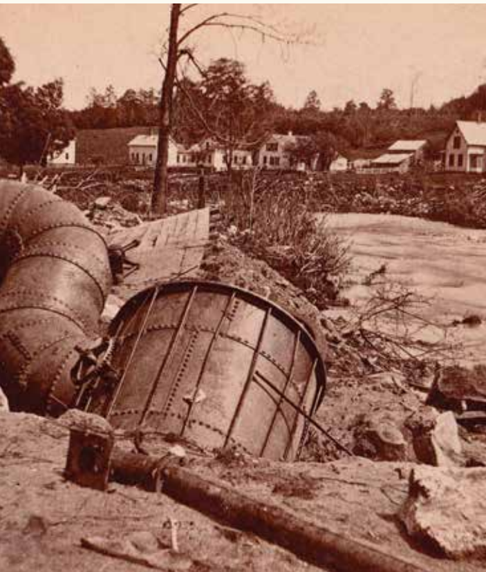
Skinner's water turbine, seen here, and the flywheel for his steam engine were the only pieces of his machinery too heavy to be swept away. Apart from them, his mill site was stripped bare.
